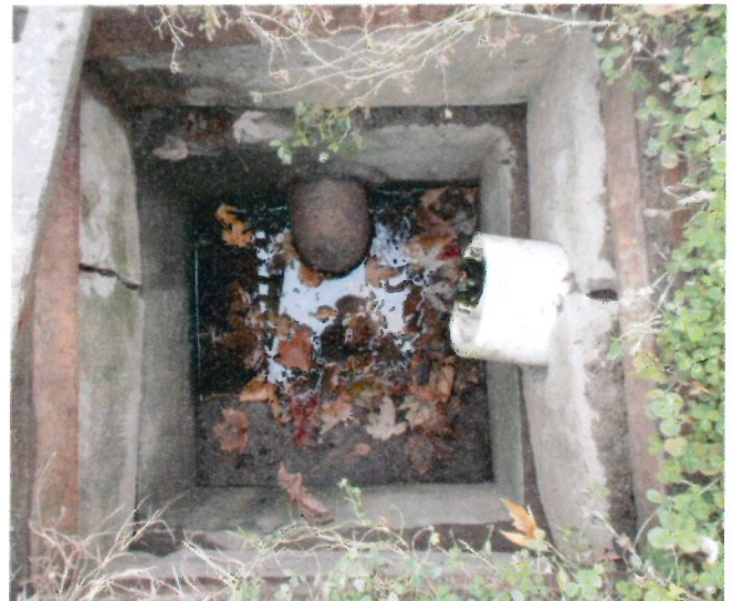
Replace existing storm water dry wells and associated underground piping at 5 locations on the west side of campus
