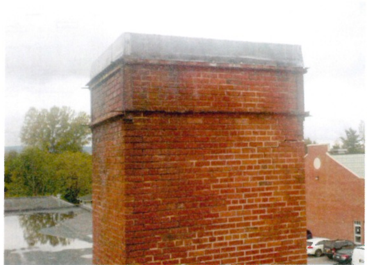
Replace deteriorated boiler chimney stack in the 1956 wing with custom flue liner
